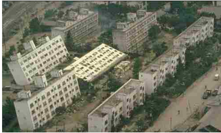
Figure 3-21: Apartment buildings after the 1964 Niigata, Japan earthquake.
